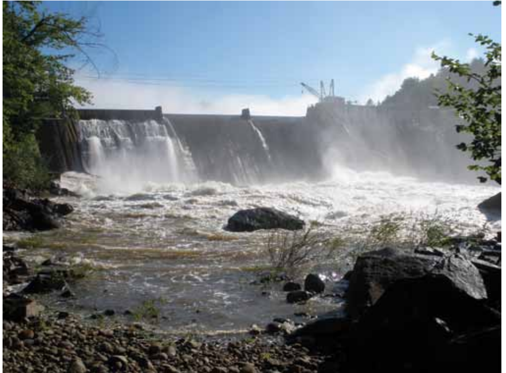
Pemigewasset River at the Ayers Island hydroelectric dam in Bristol, two days after Irene.
